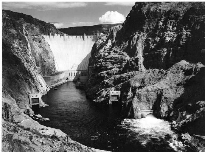
The Hoover Dam in 1941. Ansel Adams Photographs of National Parks and Monuments, Department of the Interior.
